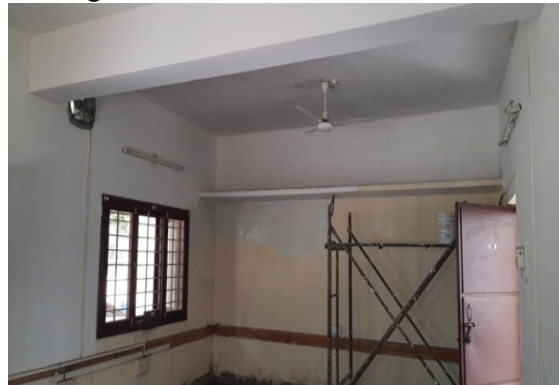
School Computer Lab (School ground floor) is being renovated.
