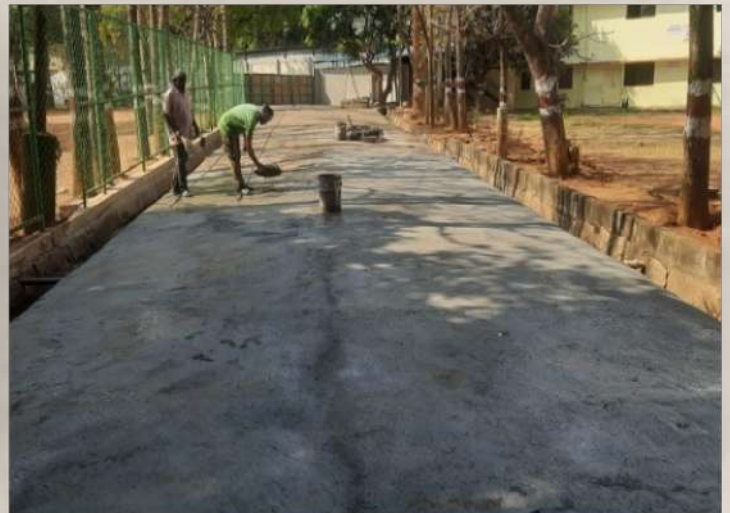
Internal road repair work
