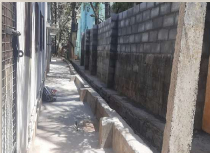
Old age home repair and maintenance done. Compound wall height raised
